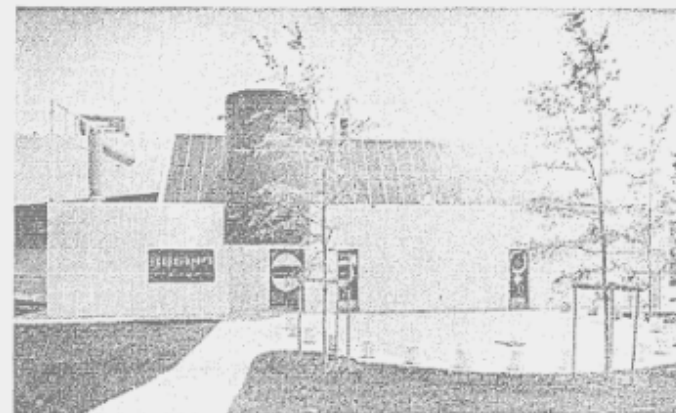
A skylight running the length of the building is the outstanding feature of the new recreation center in the Poppleton area of the city. Skylight serves to light both the upper and lower levels.
