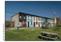
The Sarah Ann Alley houses in Poppleton, designated an "endangered building type" in Baltimore, are slated for demolition.
