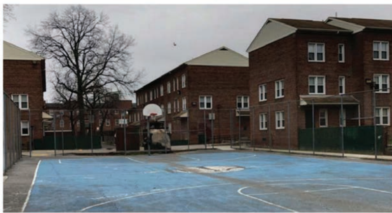
BASKETBALL COURT (PRIOR TO RESURFACING)
